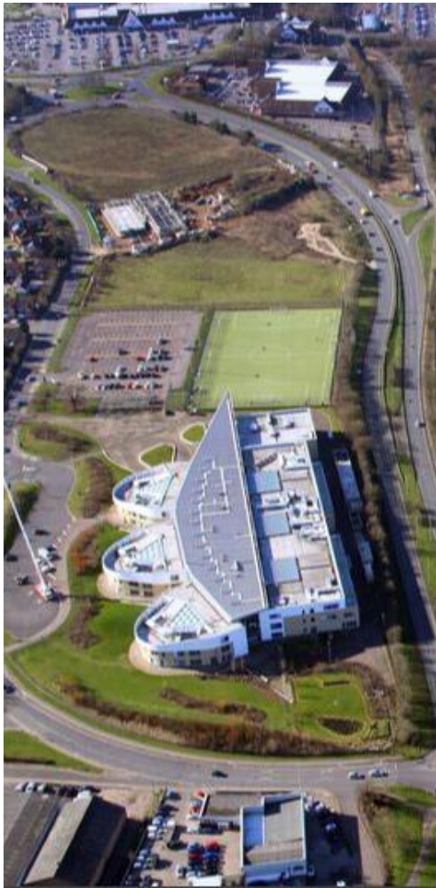
London Road, Ipswich Project
